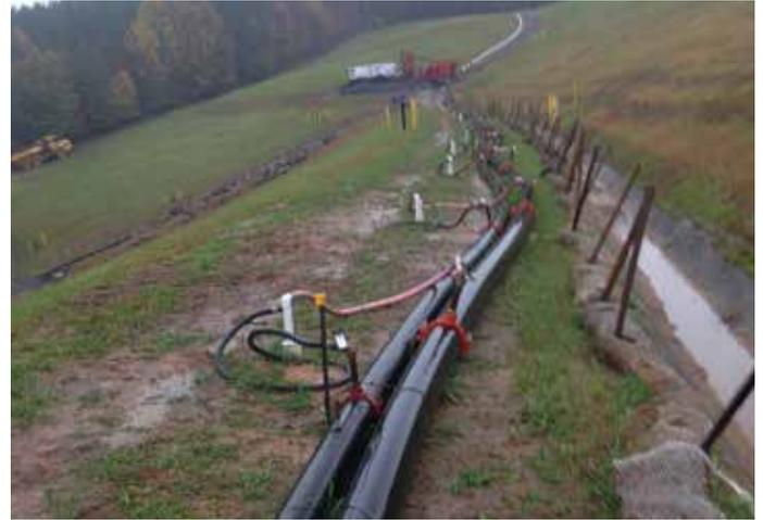
The power of pressure drives success. As high pressure water is pumped into the wells, groundwater is removed.
