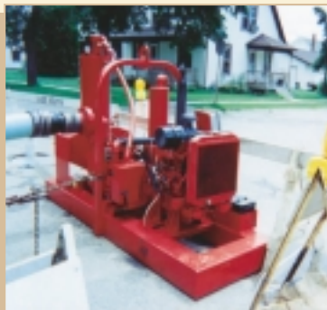
6NHRD 6" Non-Clog Pump used for a bypass operation in Janesville, Wisconsin
